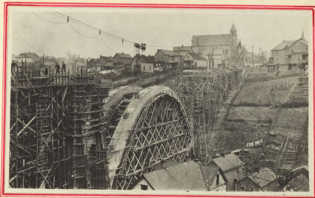
General View Showing Approach Forms and Cableway.
