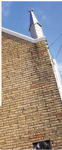
Former St. Luke's Finnish Church on Reed Ave.
